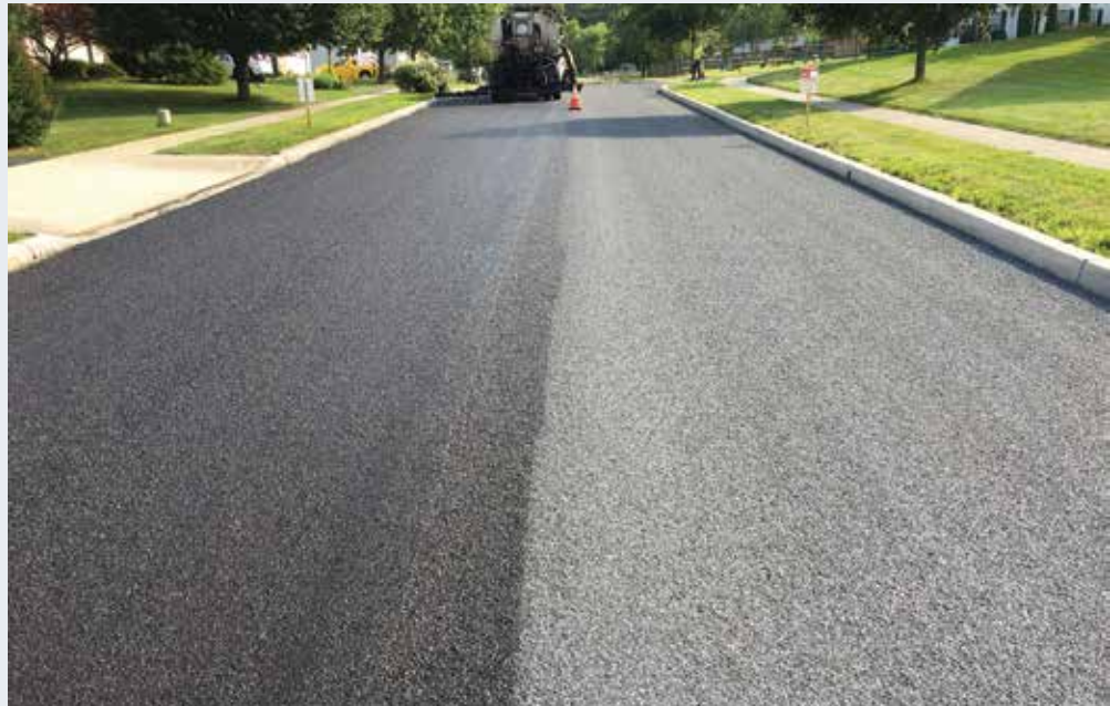
TOP: A fog seal — a thin layer of asphalt emulsion — is sprayed onto a road that has been chip sealed.
