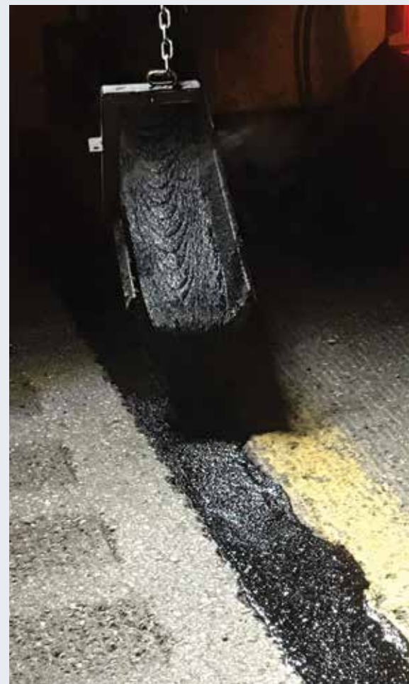
The Federal Highway Administration says filling cracks is the most cost-effective preventive maintenance tool townships can use on their roads. (Photo courtesy of SealMaster.)
